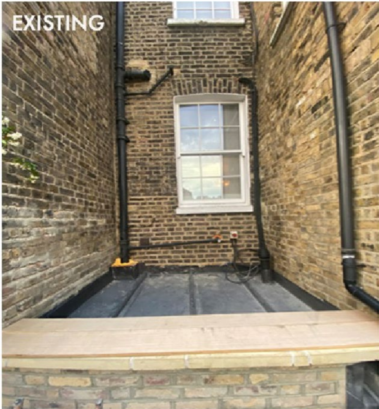
Photograph of first floor flat roof
